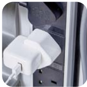
Device adaptors plug into 2 x 8-way powerstrips.
